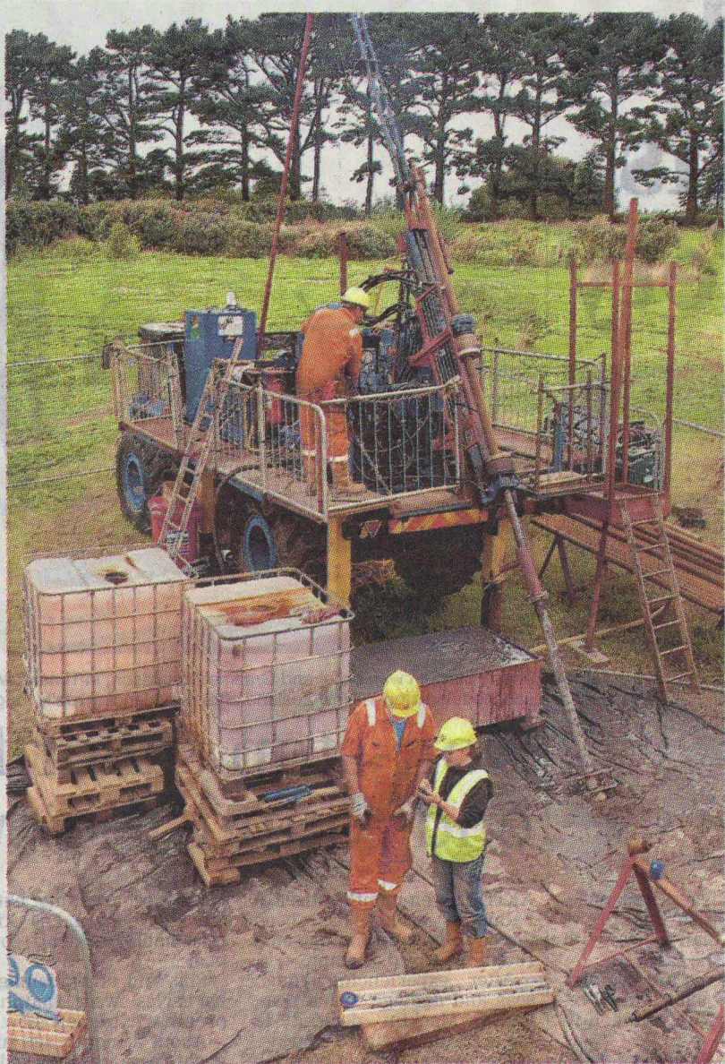
Surface drilling has begun at Duchy College Rosewarne.
